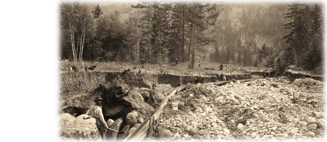
Figure 3. Linear tailings piles (at right) generated by Chinese immigrant miners using ground sluicing techniques near North Bend, Washington around 1890 (City of Vancouver Archives Item: CVA 1376-375.24).
